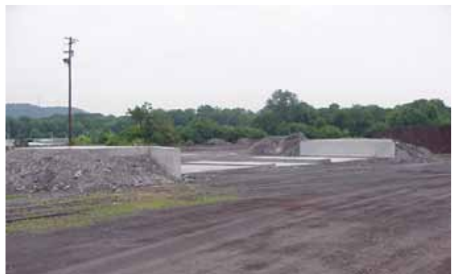
Figure 2 is the new foundation, ready for the scale installation
