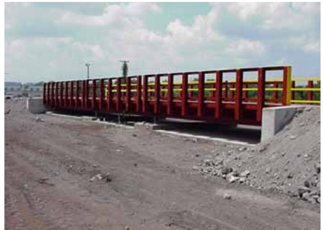
Figure 5 is finished scale, installed with attached sight rails.
