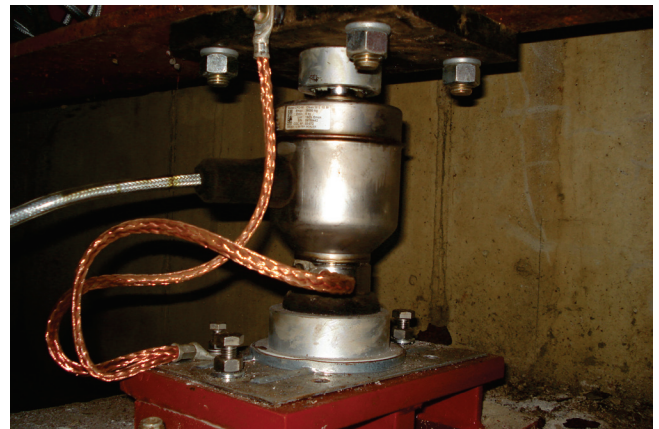
Figure 5 close up of load cell
